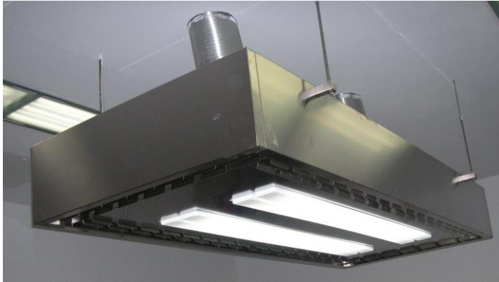
Fresh air hood with fluorescent lighting
