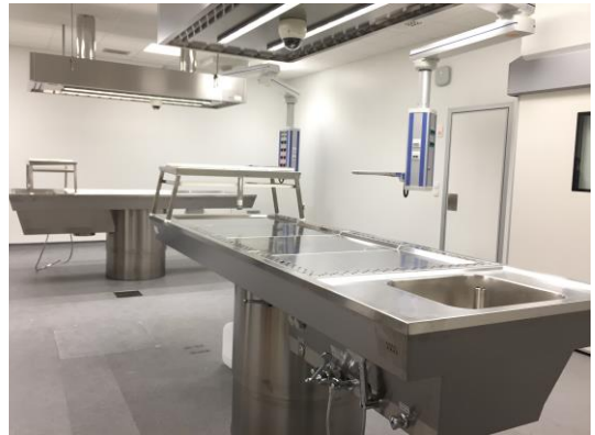
Fresh air hood with LED recessed luminaires and video camera (customized solution)
